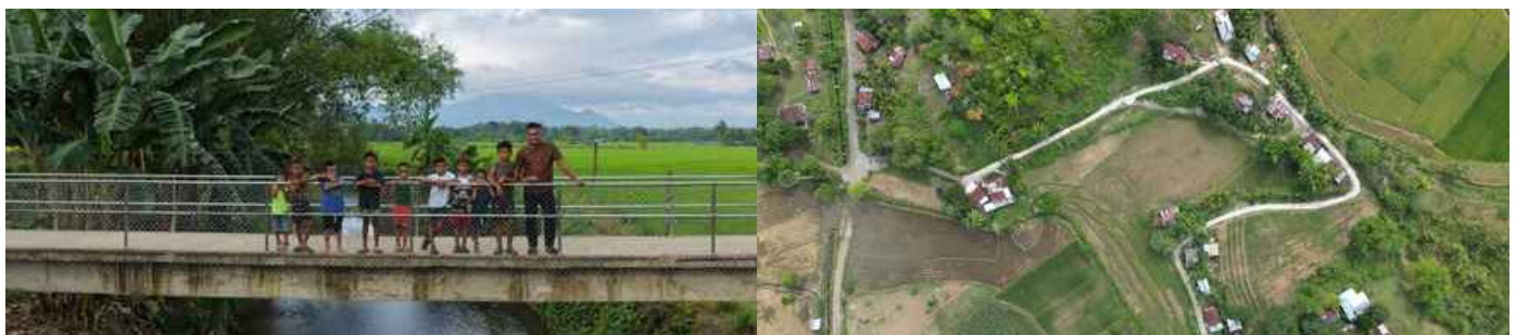
KALAHI CIDSS FOOTBRIDGE BARANGAY LOWER LANDING, DUMINGAG, ZAMBOANGA DEL SUR
